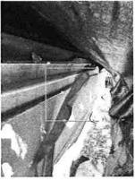
The gutter has been damaged and is no longer properly secured to the roof.
