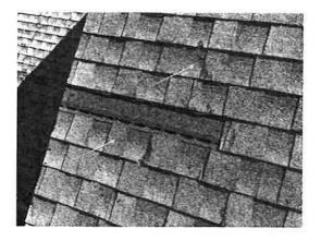
The condition of the shingles roof is poor, characterized by noticeable scratches and several missing shingles.
