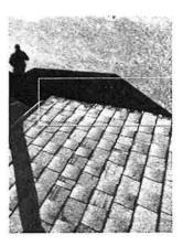
The condition of the shingles roof is poor, characterized by noticeable scratches and several missing shingles.
