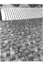
The condition of the shingles roof is poor, characterized by noticeable scratches on several areas.
