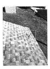
The condition of the shingles roof is poor, characterized by noticeable scratches on several areas..
