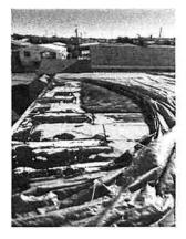
The roof is currently missing its membrane, which is a critical component for water protection and insulation.
