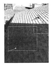
The condition of the shingles roof is poor, characterized by noticeable scratches and several missing shingles.
