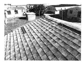
The condition of the shingles roof is poor, characterized by noticeable scratches and several missing shingles.
