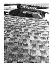
The condition of the shingles roof is poor, characterized by noticeable scratches on several areas.
